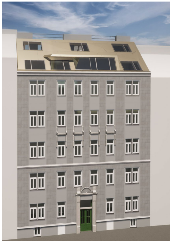
1030 VIENNA, STEINGASSE 38 MIDDLE APARTMENT HOUSE / OPTIMISATION OF EXISTING BUILDING / STUDY APPROX. 805 M 2 OF EXISTING SPACE + 210 M 2 OF ATTIC EXTENSION PURCHASE: Q1 2021 SALE: Q4 2021
